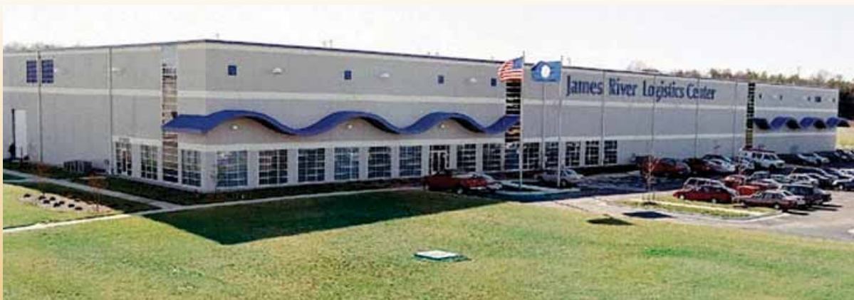
James River Logistics Center at 812,000 square feet is representative of the distribution facilities found in Chesterfield County and the region.
